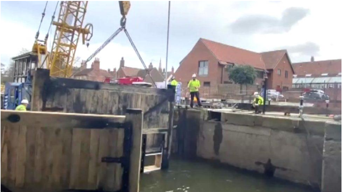
Newark Town lock gate replacement (CRT)
