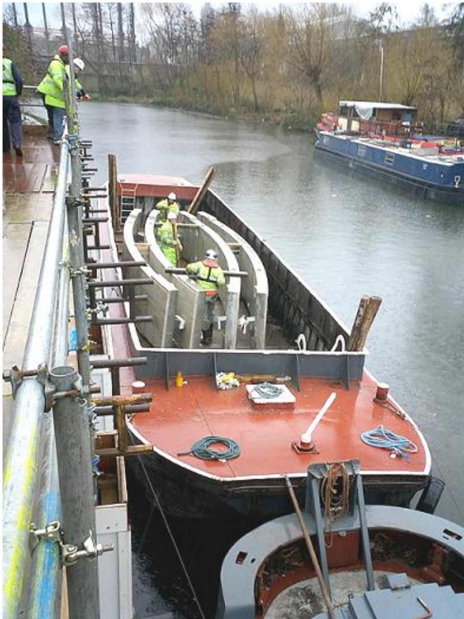
Tunnel linings being transported (WHH)
