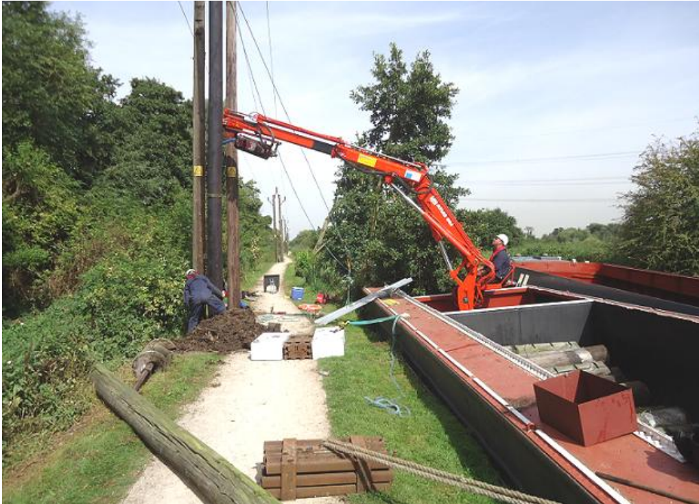
Installing electric poles on the River Lee (WHH)
