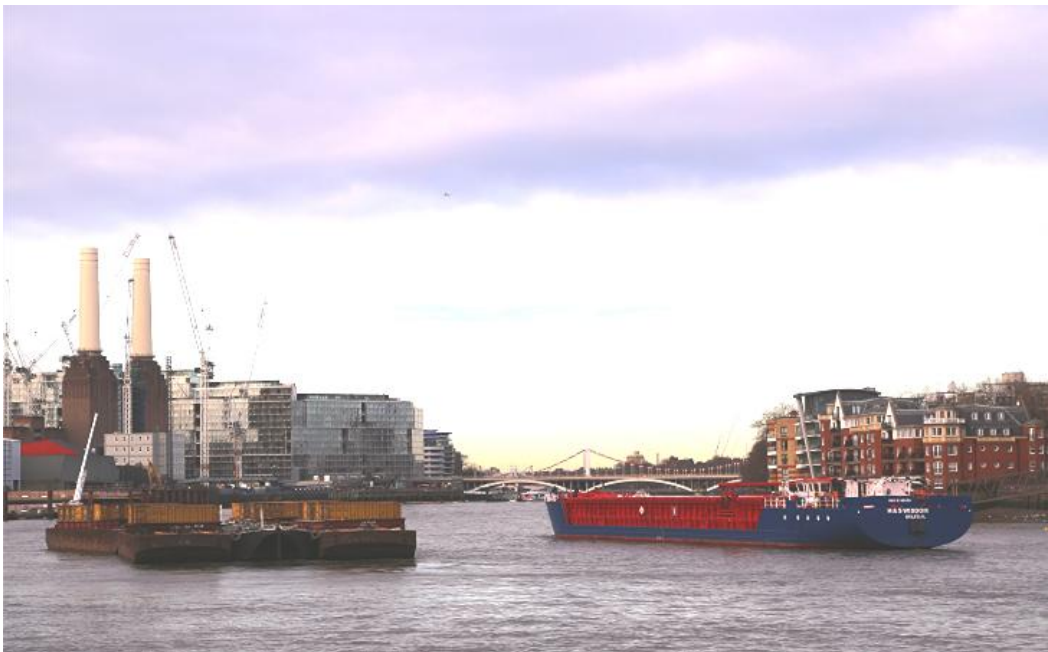
Arrival of tunnel boring machines named Millicent and Ursula for the Tideway Tunnel (Tideway)
