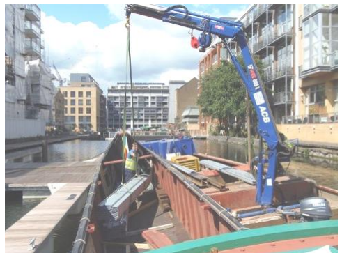
Arundel unloading piles at Kingsland Basin (R. Horne)
