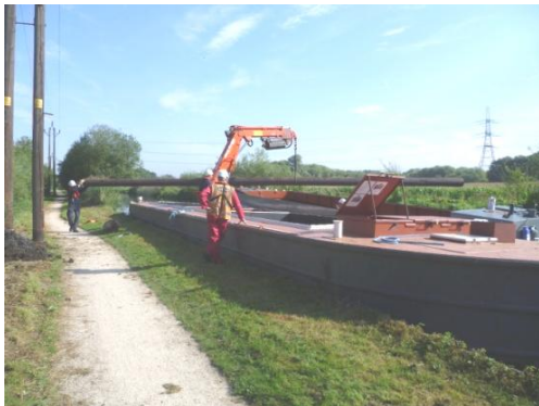
WHH hopper, and barge Everton unloading poles (WHH)
