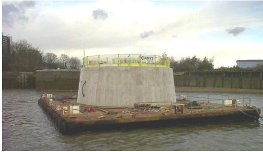
Pontoon Dart with 400 tonne concrete unit (Livett's)
