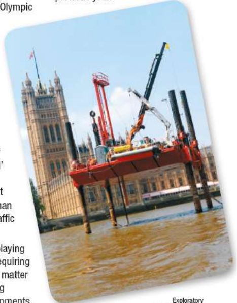
Exploratory works taking place in the riverbed outside the Palace of Westminster, where a borehole has been sunk from a large rig to analyse the ground conditions that engineers digging the proposed Thames Tunnel are likely to encounter. © Wessex Water
